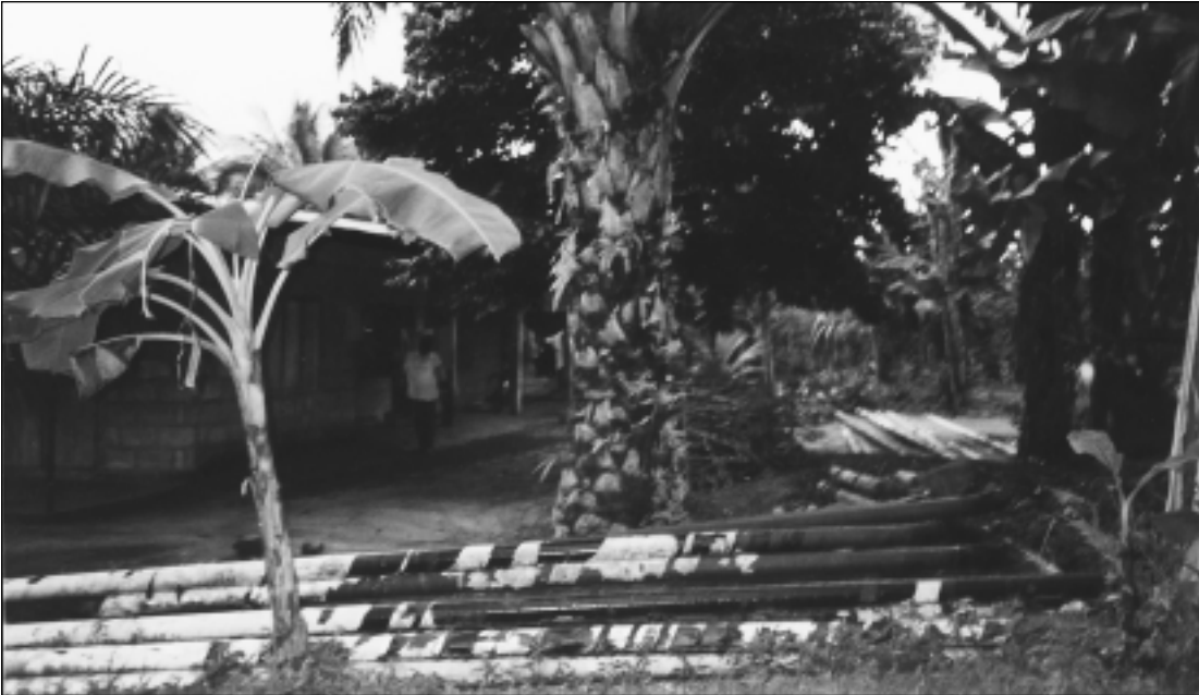
Pipelines crossing a yard in the Ogoni village of K-Dere, Rivers State. (Photo: Eowyn Greeno)
